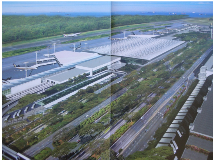
Overall view of the Terminal 3 after finished
