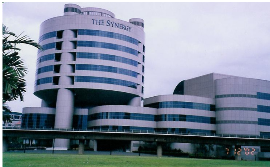
Synergy Building, Singapore
